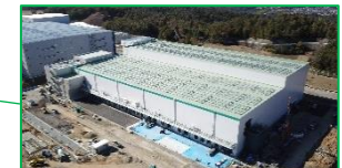
HN new Minoh-Shinmachi branch (under construction)
